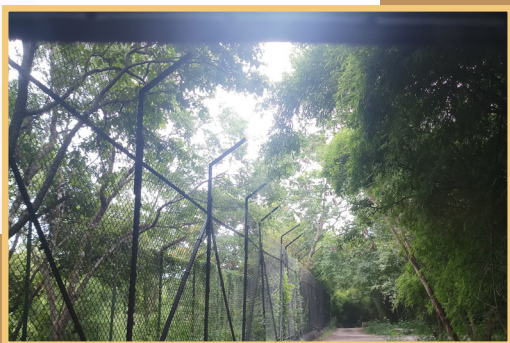
Strengthening of chainlink fencing at safari
